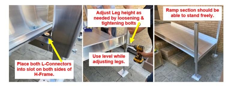
Step 7: On the remaining Ramp sections repeat Steps 4 & 6 as shown below.
